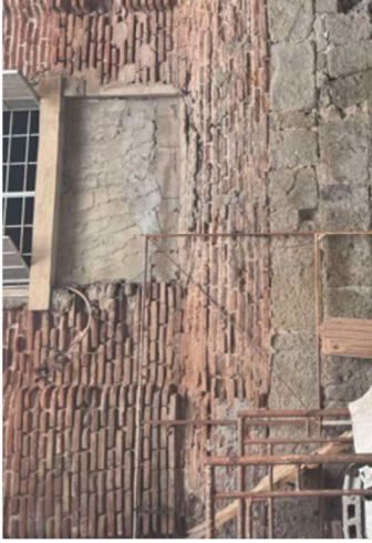
REPAIR OF MISSING BRICKS ON WALL
